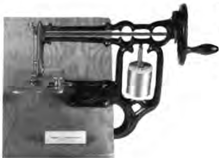
Figure 93.—HANCOCK SEWING MACHINE, 1867. One of the many inventors who turned his talents to inventing and producing a mechanically simple and cheaper machine was Henry J. Hancock. His 1867 machine is only about six inches wide; it uses a tambour-type needle, pulling a loop of thread from below the stitching surface. (Smithsonian photo P63197.)
