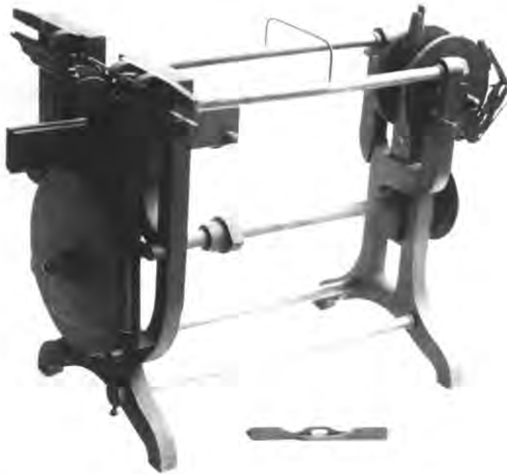
Figure 13.—CORLISS' PATENT MODEL, 1843. The piece of wood in the foreground is an enlarged model of the needle. (Smithsonian photo 42490.)
