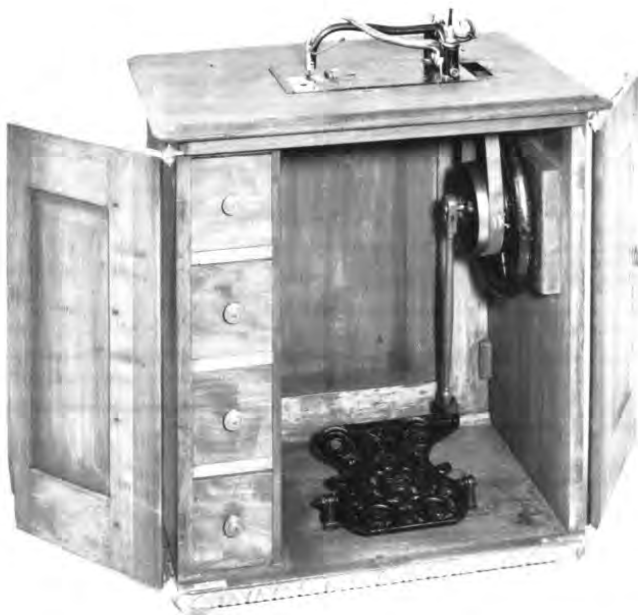
Figure 35.—THIS GROVER AND BAKER CABINET-STYLE SEWING MACHINE of 1856 bears the serial number 5675 and the patent dates February 11, 1851, June 22, 1852, February 22, 1853, and May 27, 1856. (Smithsonian photo 45572-F.)
