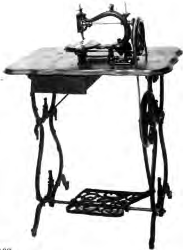
Figure 148.—THE SECOR LOCK-STITCH SHUTTLE SEWING MACHINE as illustrated in a broadside of about 1870. The name of the sewing-machine company cast into the treadle, or some other part of the framework, became increasingly common. (Smithsonian photo 67219.)
